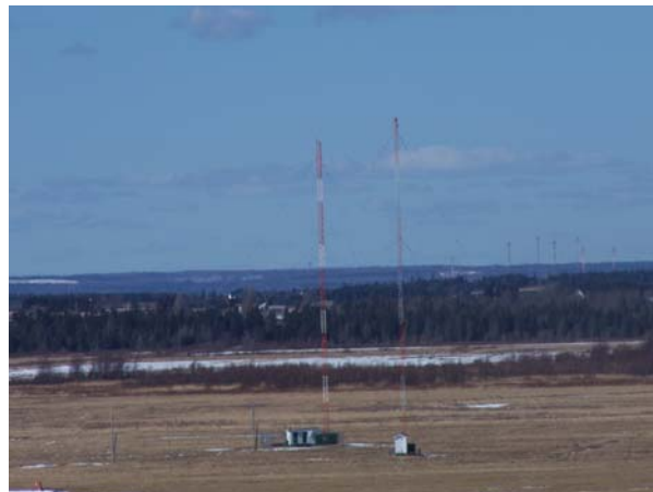
Figure 3.4. Image of the AM radio towers
